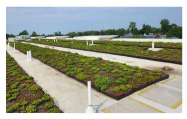
An otherwise unused space, the rooftop of a Philadelphia four level multifamily asset has been converted to a green roof aimed at improving sustainability. The roof i) reduces stormwater runoff, ii) cools the roof surface, improving energy efficiency, iii) increasing biodiversity (wildlife such as bees and butterflies), and iv) absorbs carbon dioxide and pollutants.
