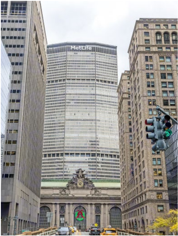
MetLife Building, New York
